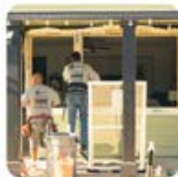
WINDOWS AND DOORS
